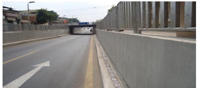
Tunnel in Giza
